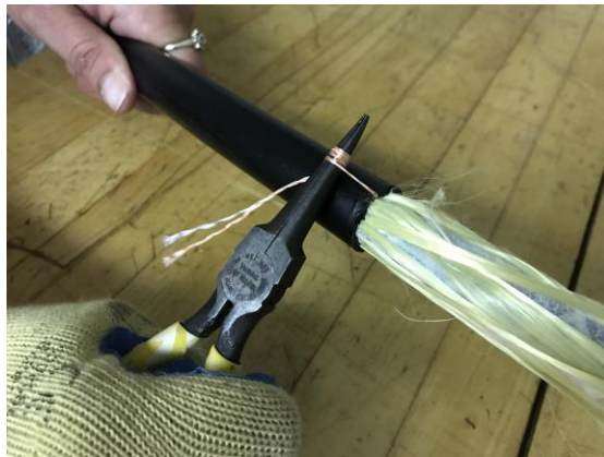
Figure 7 – Pull the rip cord through the outer jacket.
