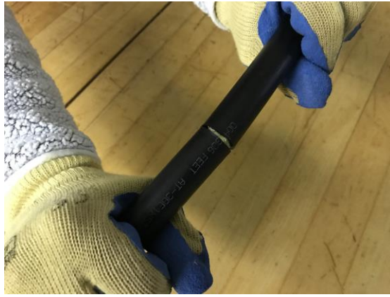
Figure 5 – Flex the cable to open the ring cut.
