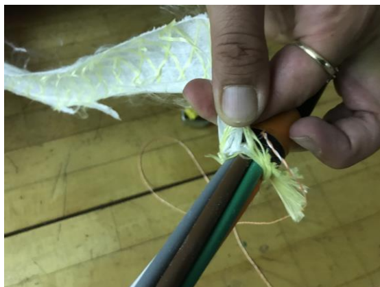
Figure 19 – Remove binder threads and water blocking tape.
