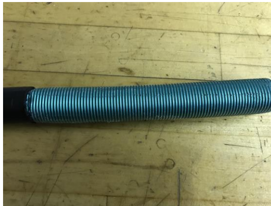
Figure 27 – Remove the outer jacket to expose the armor tape.
