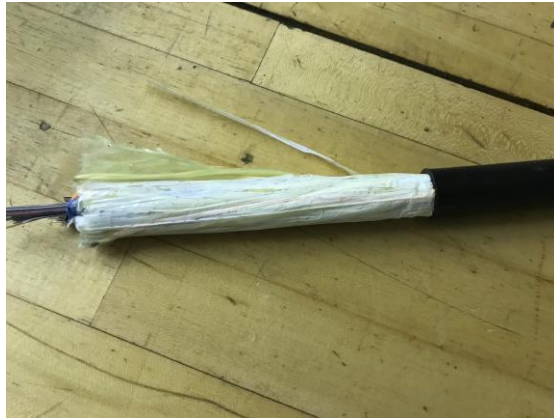
Figure 6 – Remove the 6 inch piece of outer jacket.
