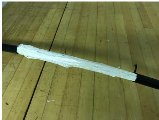
Figure 15 – Open a 10 inch window in the middle of the cable.
