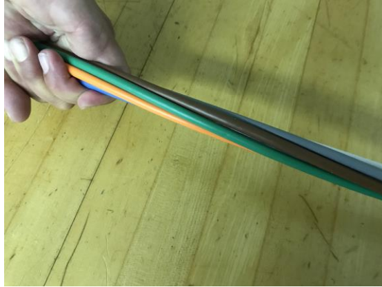
Figure 20 – Unwind the buffer tubes from the strength member.
