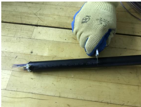
Figure 3 -- Ring cut the cable 6 inches from the end.
