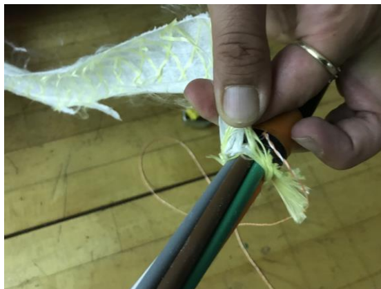
Figure 10 – Remove binder threads and water blocking tape.
