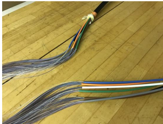
Figure 26 – Remove the tubes from the fibers.
