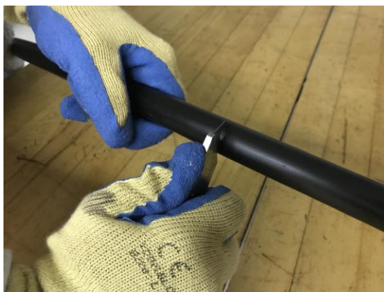
Figure 4 – Ring cut the cable at required length.
