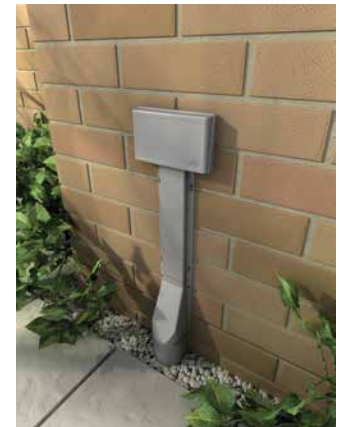
Installed External CSP Module
