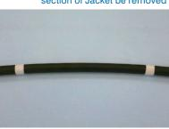
STEP 4: Cut around the cable at the both ends (Circular)
