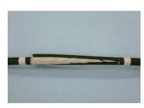
**STEP 3 :** Cut the cable laterally between the marked position.
